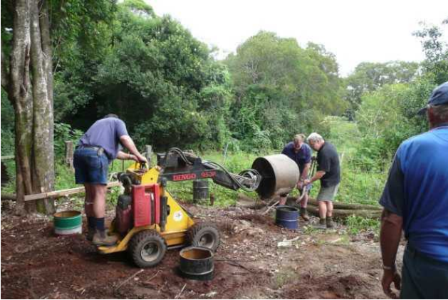
Preparing the Site
